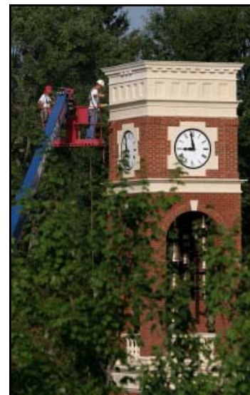
Workers put finishing touches on the top of the new Carillon.
