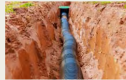
Repair and Replace Campus Water Lines $3,500,000
